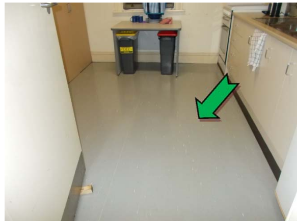
Photo 4. Interior, kitchen, floor coverings – suspected non asbestos-containing vinyl sheet.
