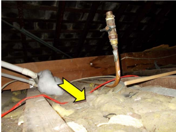
Photo 7. Interior, ceiling space, insulation – suspected SMF insulation batts.
