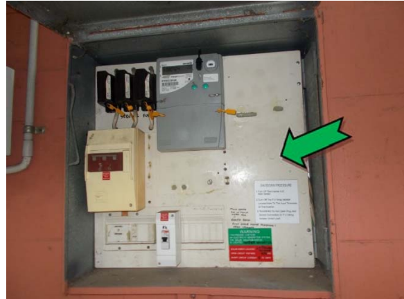
Photo 2. Exterior, south elevation, electrical board – suspected non asbestos-containing bituminous backing board.
