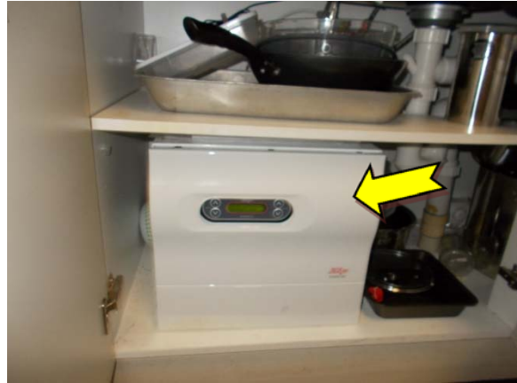
Photo 8. Interior, kitchen, hot water heater – suspected SMF internal insulation material.
