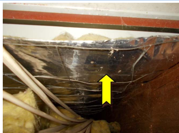
Photo 6. Interior, ceiling space, insulation – suspected SMF sarking insulation material.
