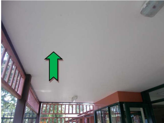
Photo 1. Exterior, throughout, awning – non asbestos-containing fibre cement sheeting.
