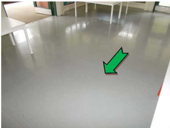
Photo 3. Interior, main room, floor coverings – suspected non asbestos-containing vinyl sheet.
